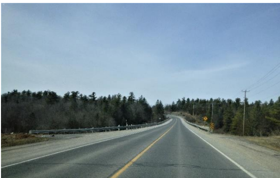
Image 1: View of Taylor Kidd Boulevard looking west towards Lake Ontario (Bay of Quinte-North Channel).
