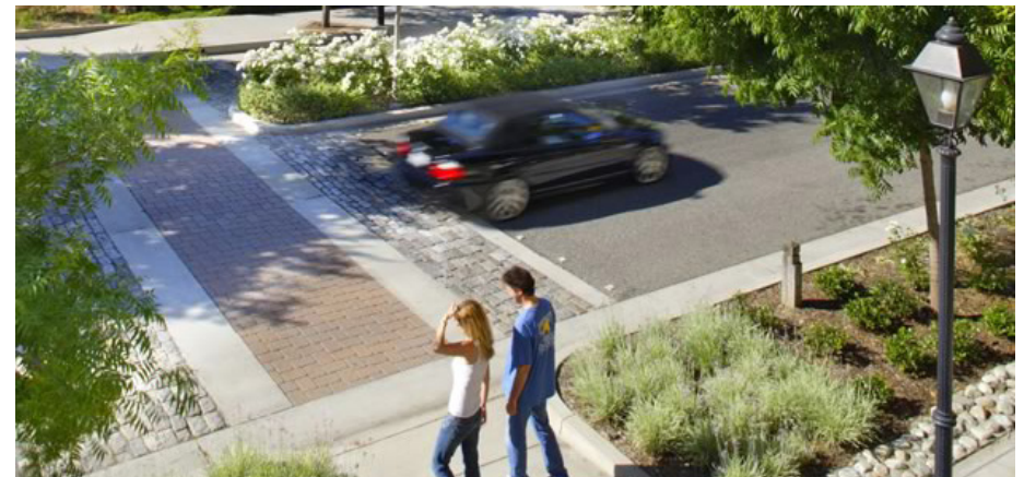
Figure 3.28 - Pedestrian Crossing as Traffic Calming Raised table crossing
