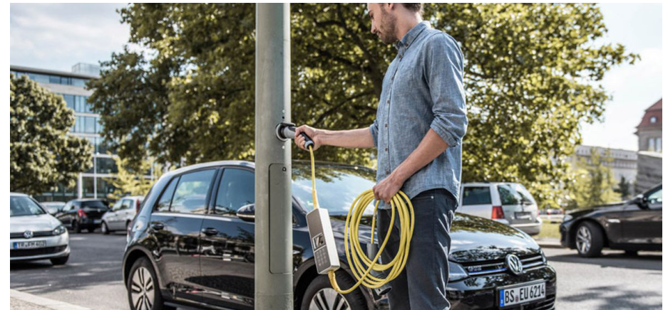
Figure 3.29 - Electric Vehicle Charging Station
