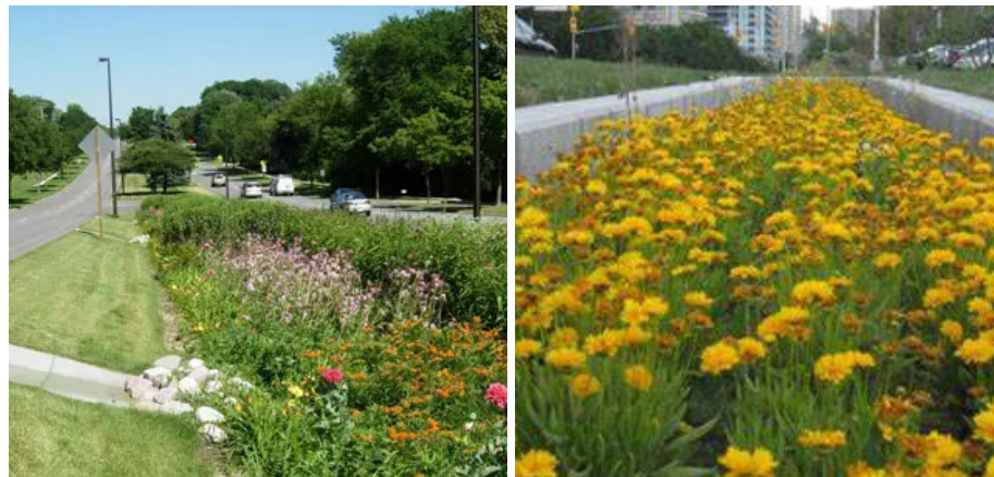
Figure 3.8 - Bioswales and Bioretention Planters Bioswale, @Parks and Recreation Magazine | Bioretention Planter, Credit Valley Conservation
